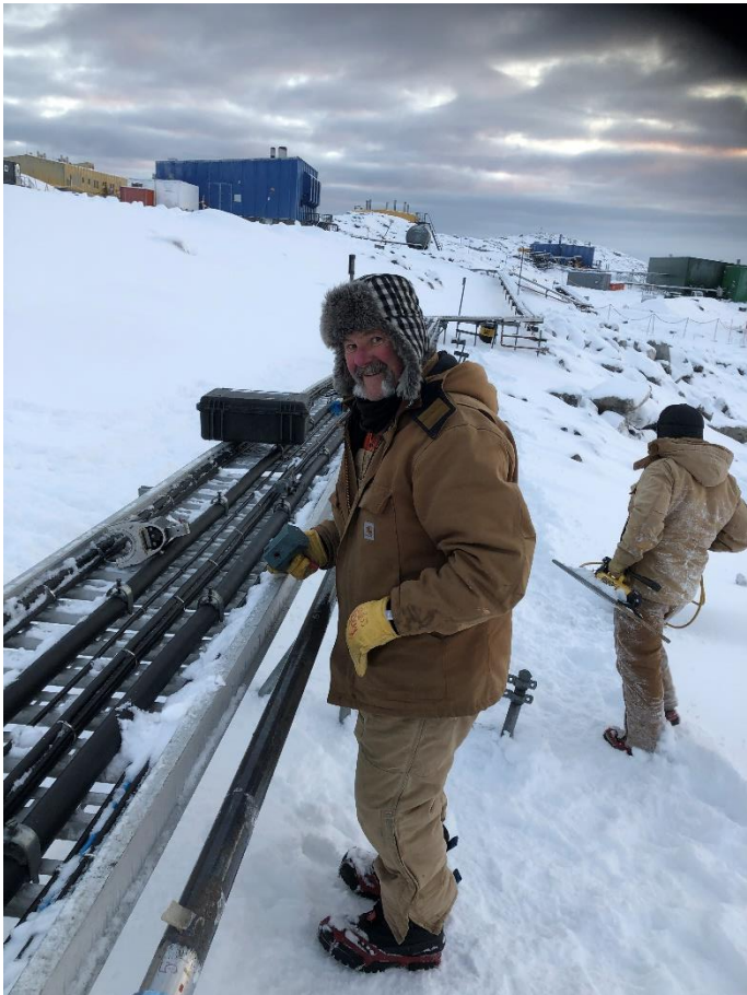
Repairs to a fuel line
